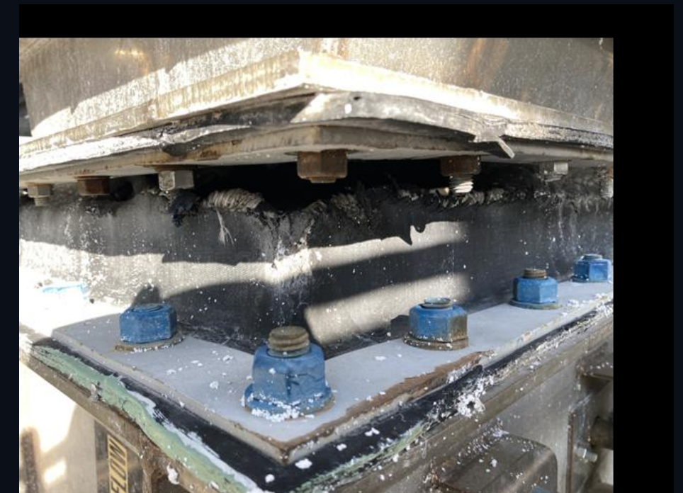
Degraded duct seals / gaps found on blower-to-dryer air lines.
